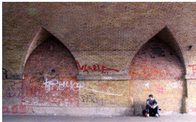
Fig 4.3.64: Photo: Current view of in-filled cross arches within listed viaduct
