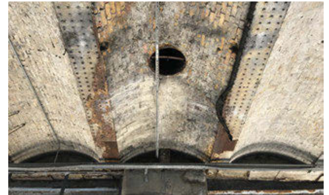
Fig 4.3.75: Photo: Current view of jack arches with Oculi opening
