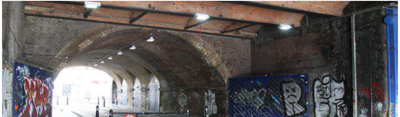
Fig 4.3.63: Photo: Current view showing jack arch, barrel vault and listed viaduct structure
